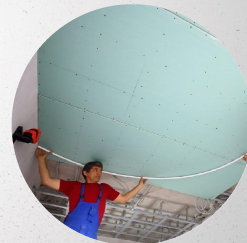
dry construction and plastering
